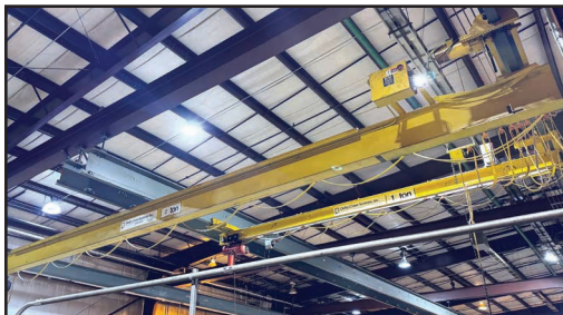
VIEW OF DELTA CRANES
