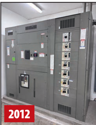
EATON POW-R-LINE SWITCHBOARD SWITCHGEAR
