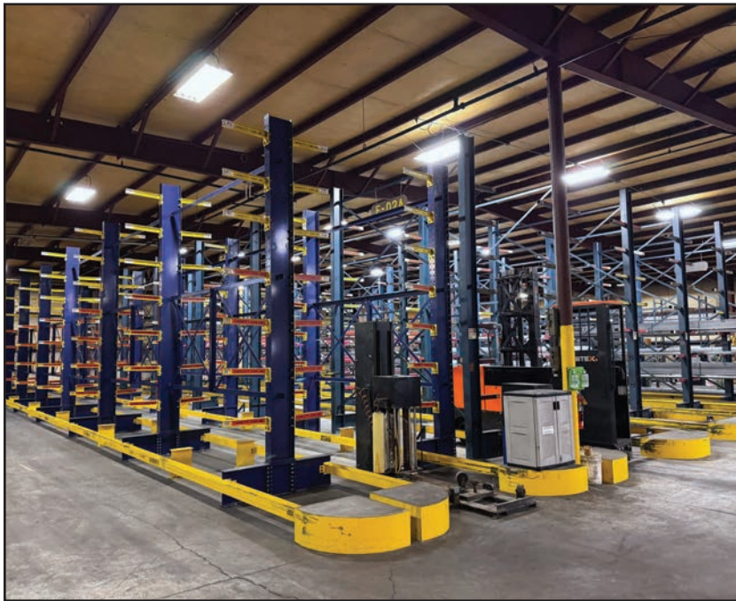
VIEW OF HEAVY DUTY CANTILEVER RACKING
